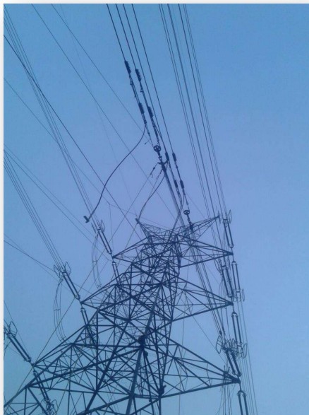
Fig-1: De-stringing work of damaged tower
