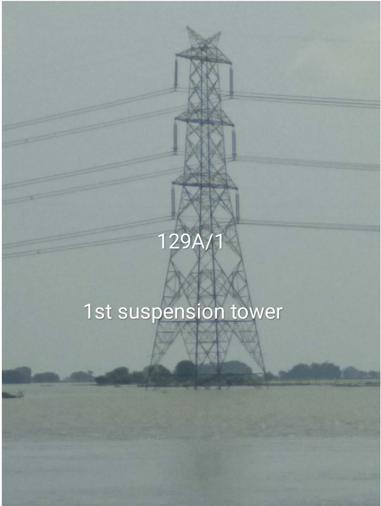
Tower at Loc. No. 129A/1
