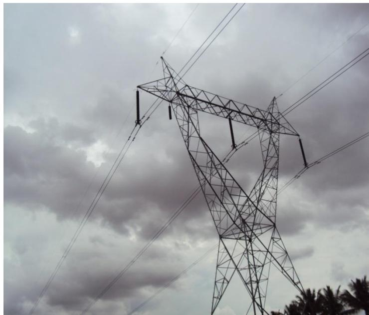
Figure: 2 Photograph showing the dummy insulators installed at identified testing tower
