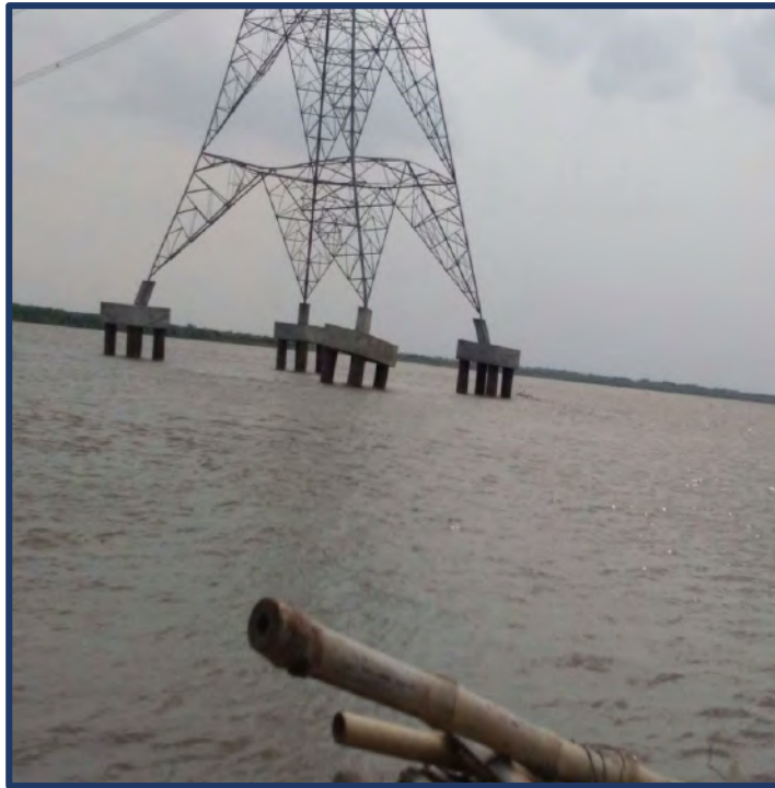
27/1 with tilted pile cap in mid stream without protection
