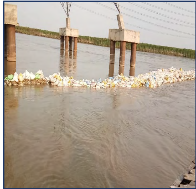
Construction of temporary C shape bund in progress to reduce water flow to avoid further damage
