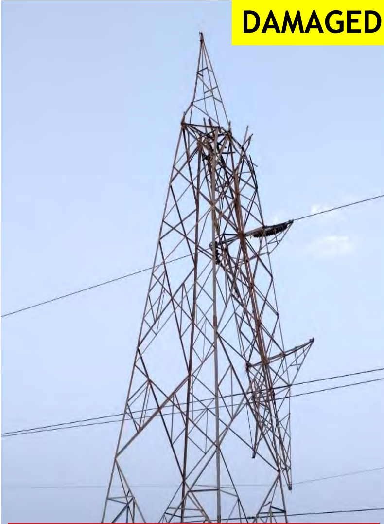
DAMAGED TOWER 220KV MENDHASAL-CHANDAKA AT LOCATION NO 35 ON 3 RD MAY
