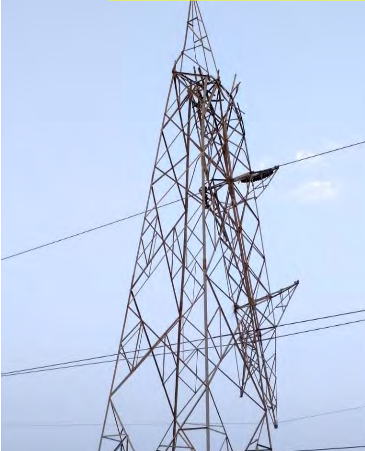
DAMAGED TOWER 220KV MENDHASAL-CHANDAKA AT LOCATION NO 35 ON 3 RD MAY
