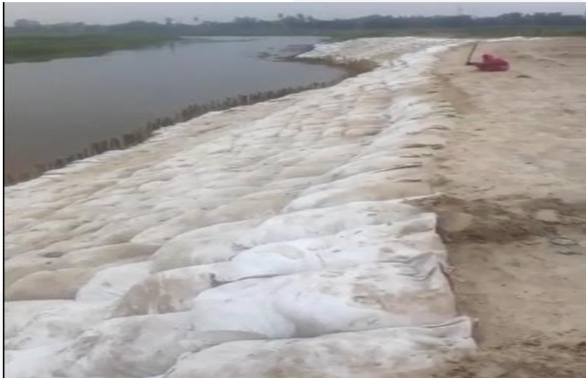
Protection of tower foundation in Darbhanga Line
