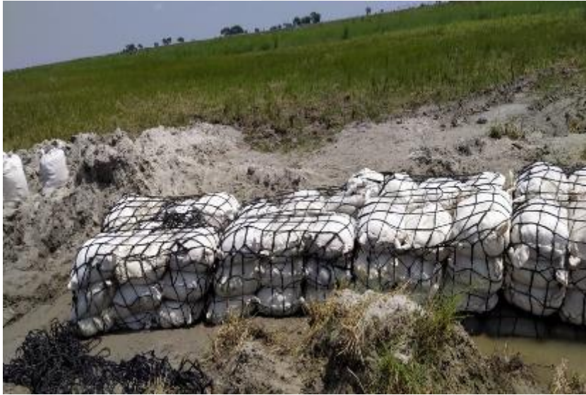
Protection of tower foundation via Gabions
