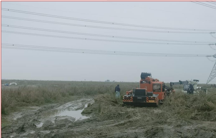
Damage done to access roads and piling location due to rain during first and second week of Mar 2020
