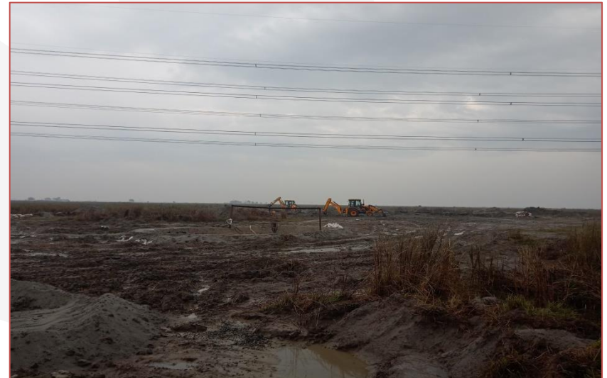
Damage done to access roads and piling location due to rain during first and second week of Mar 2020
