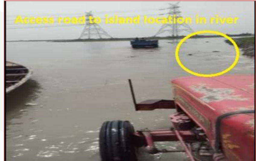
Damage done to access road for material mobilization and movement to Island loc
