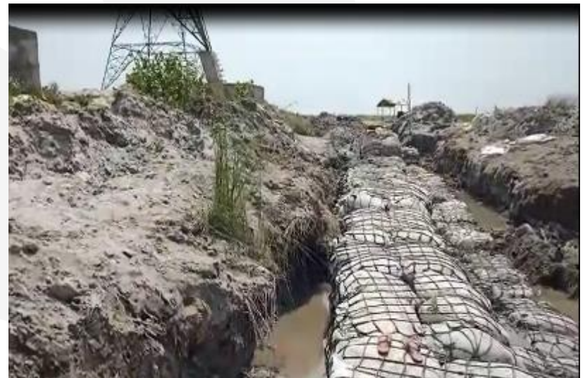
Protection of tower foundations in LIL section
