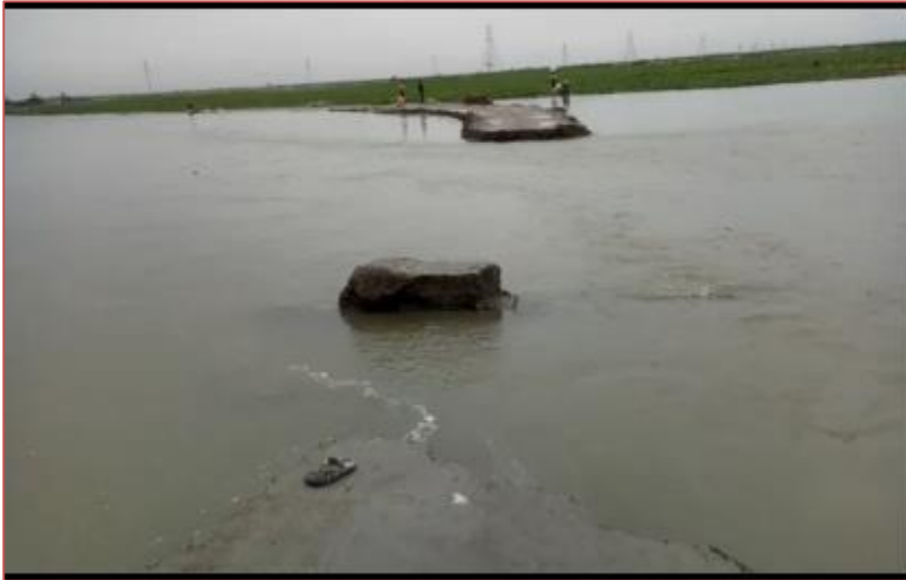
Damage done to access road for material mobilization and movement to Island loc
