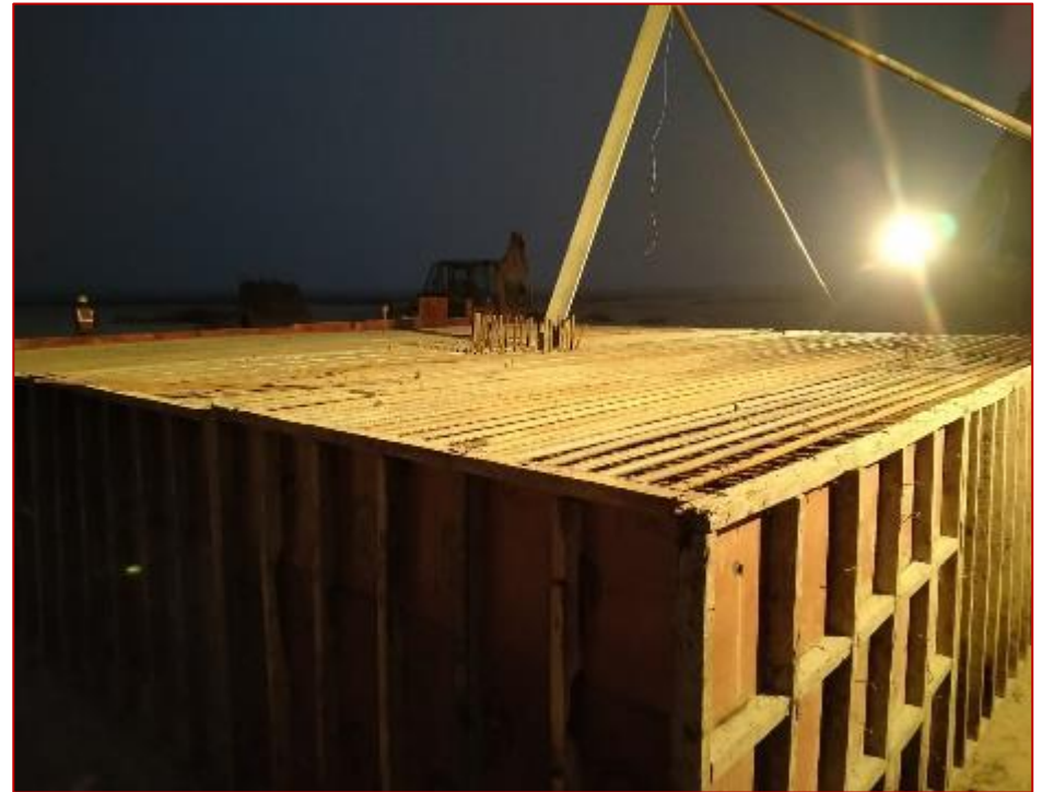
Pile cap work in progress
