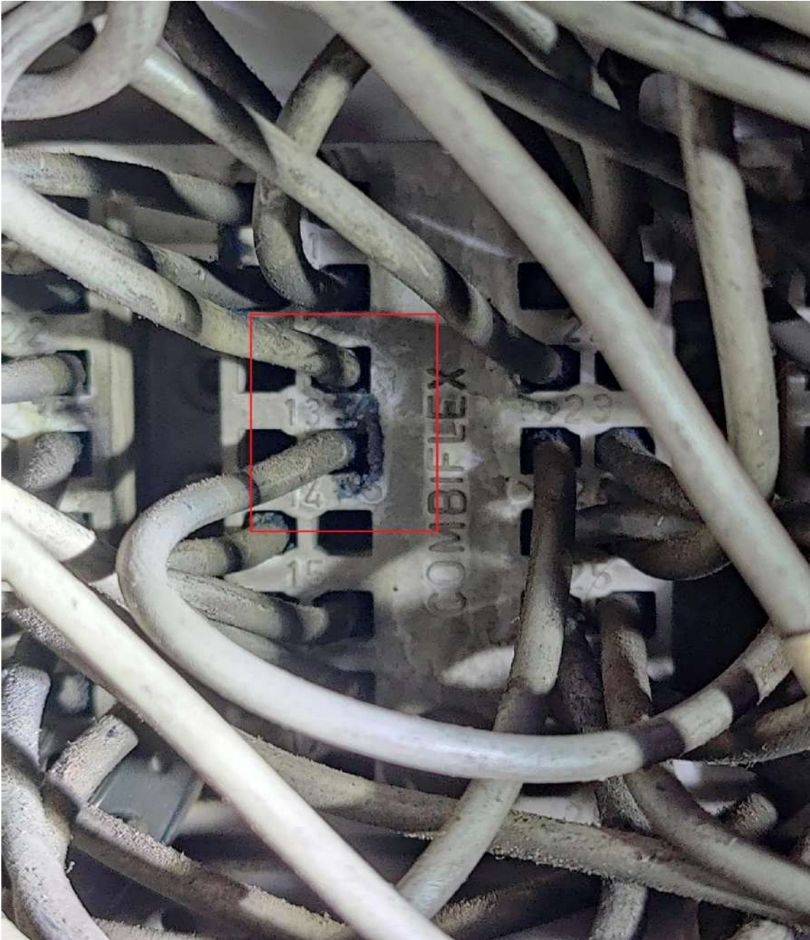
Picture 1- Relay terminal 13,14 of B phase single phase auxiliary trip relay (86B2) was found shorted through combiflex plinth.
