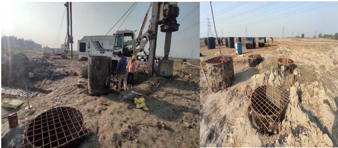
Liner driving work in progress as on 01.12.2022
