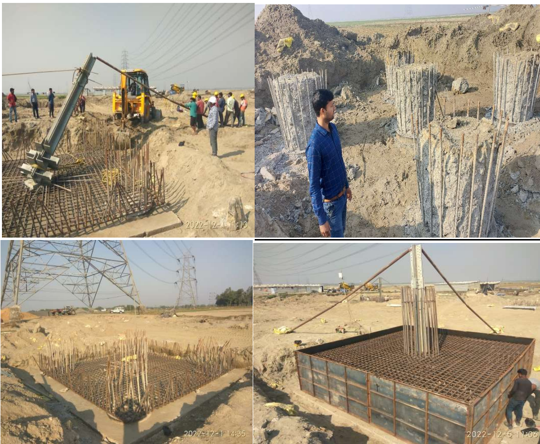
Pile Cap foundation work under progress as on 01.12.2022
