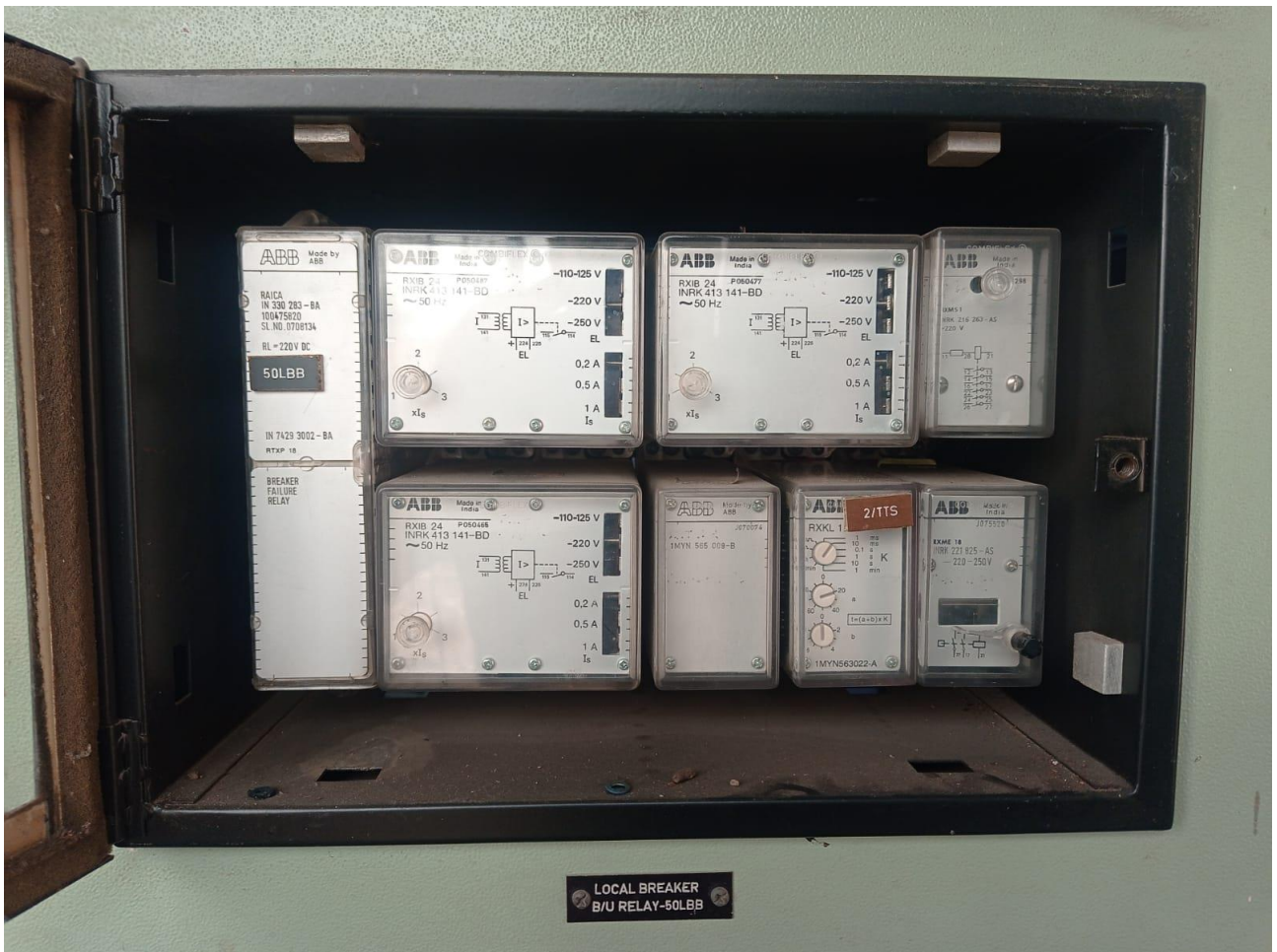
Picture 1-LBB relay iro KLC-NTAIII 220 KV circuit.
