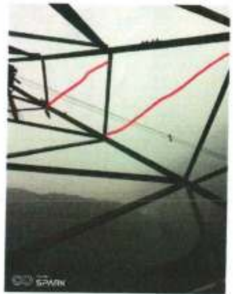
Pic 2. Missing Tower Members on T.No.49
