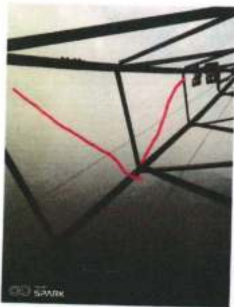
Pic 3. Missing Tower Members on T.No.49
