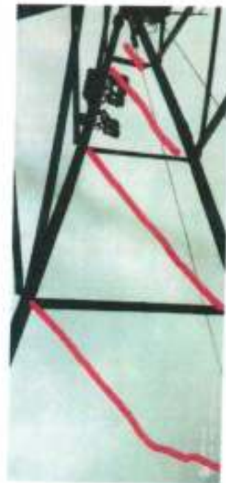
Pic 4. Missing Tower Members on T.No.49
