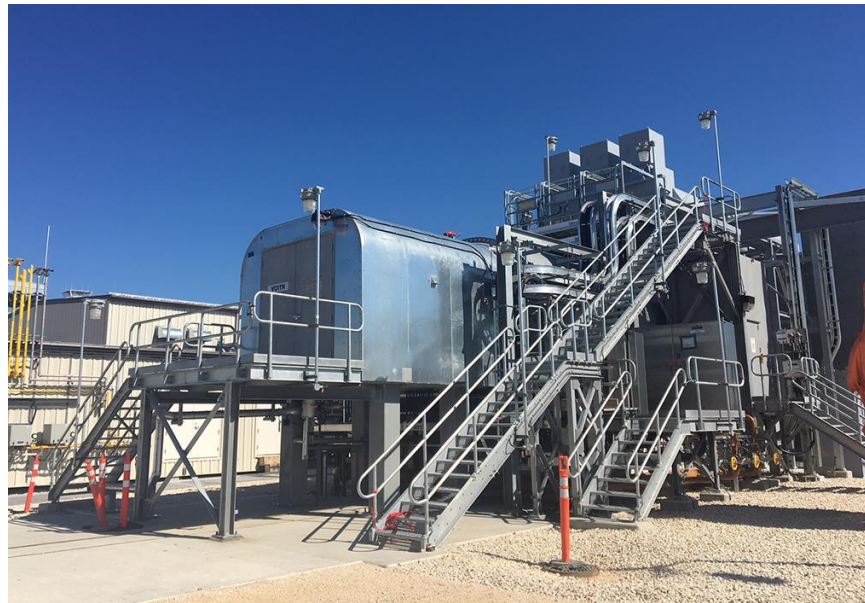
One of the four 250 MVAR synchronous condensers
