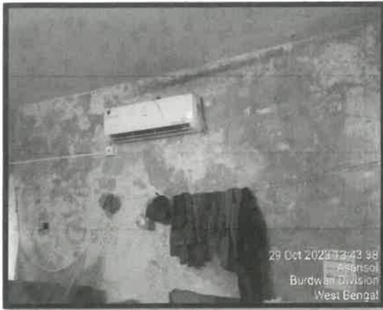
Dampness and crack with cosmetic repair in D2 quarter
