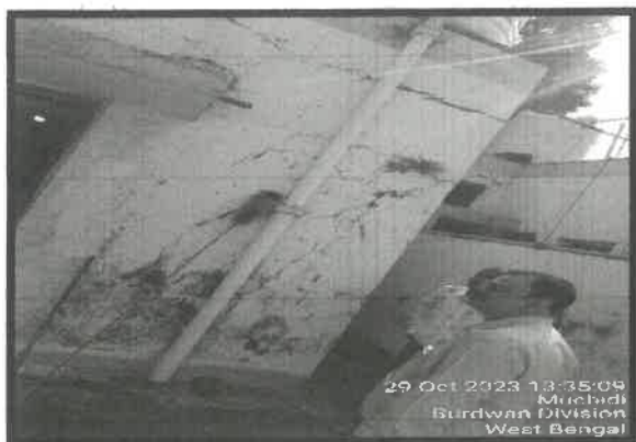
Cracks on back wall of B-quarter
