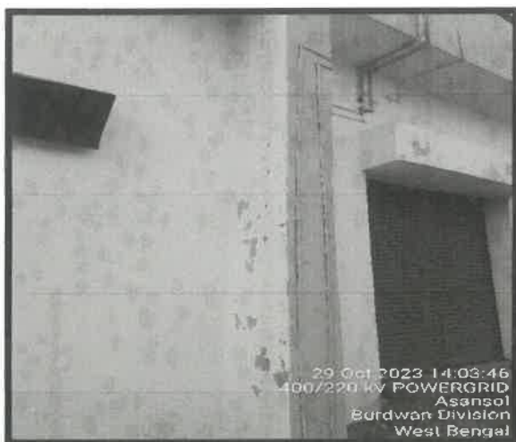
Cracks on exterior wall of control room building
