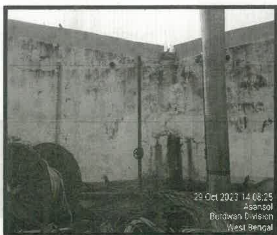
Crack line on the top of firefighting tank
