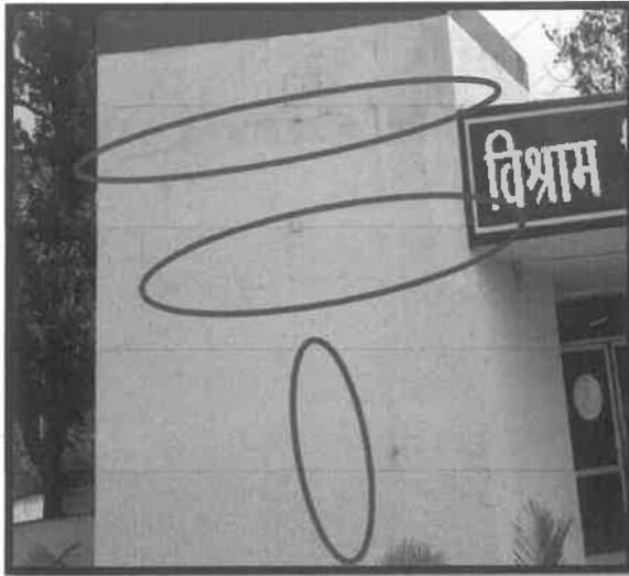
Cracks on front and back portion walls of Transit camp
