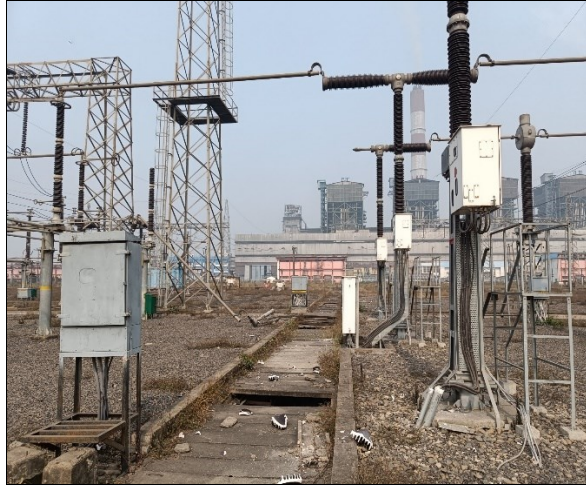
Fig. – 1 (B-Pole found to be damaged with shattering of interrupter porcelain)
