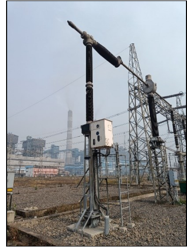
Fig. – 1 (B-Pole found to be damaged with shattering of interrupter porcelain)
