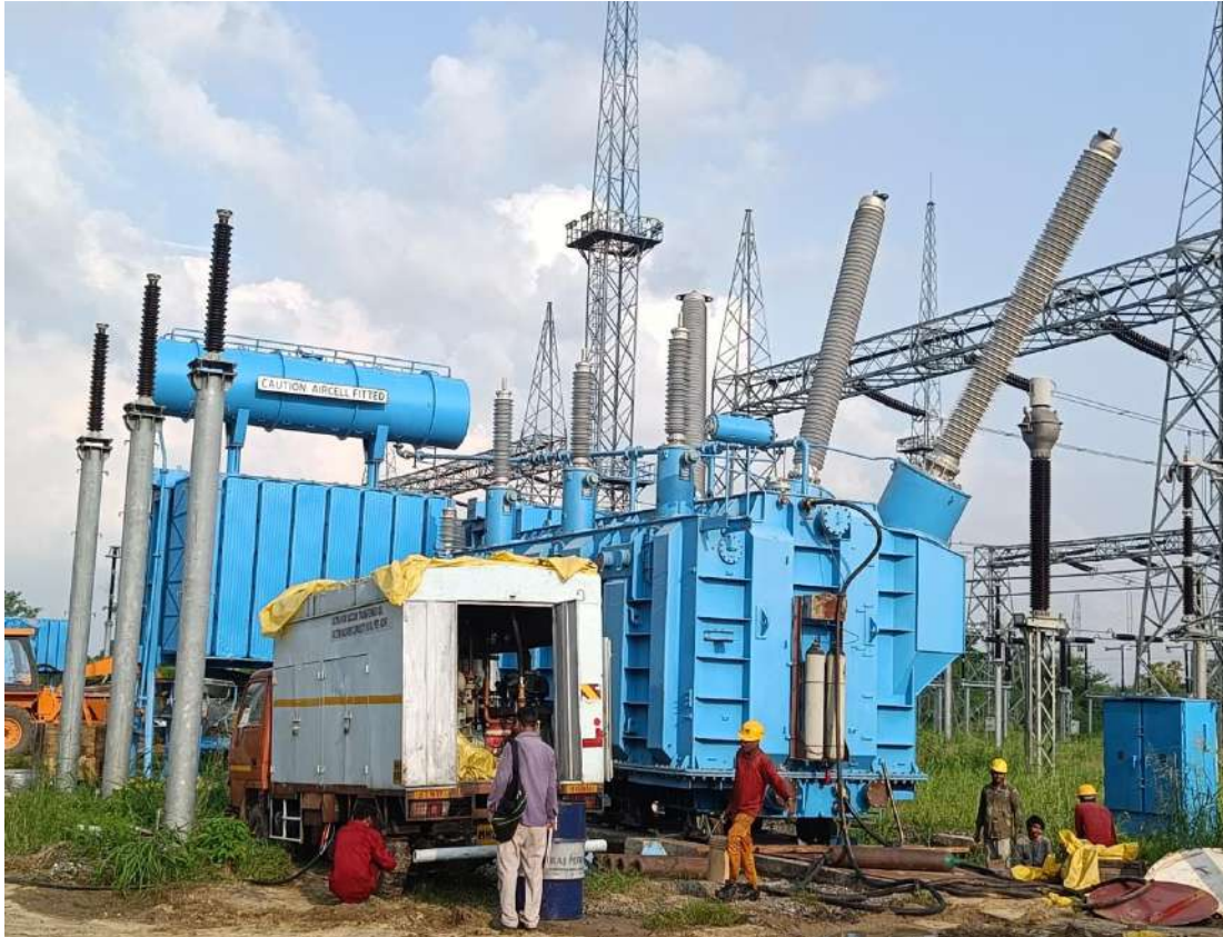
2 Nos. 200MVA ICTs Erection and Commissioning Manufacturer- BHEL FDPS – M/s GE T&D (I) Limited
