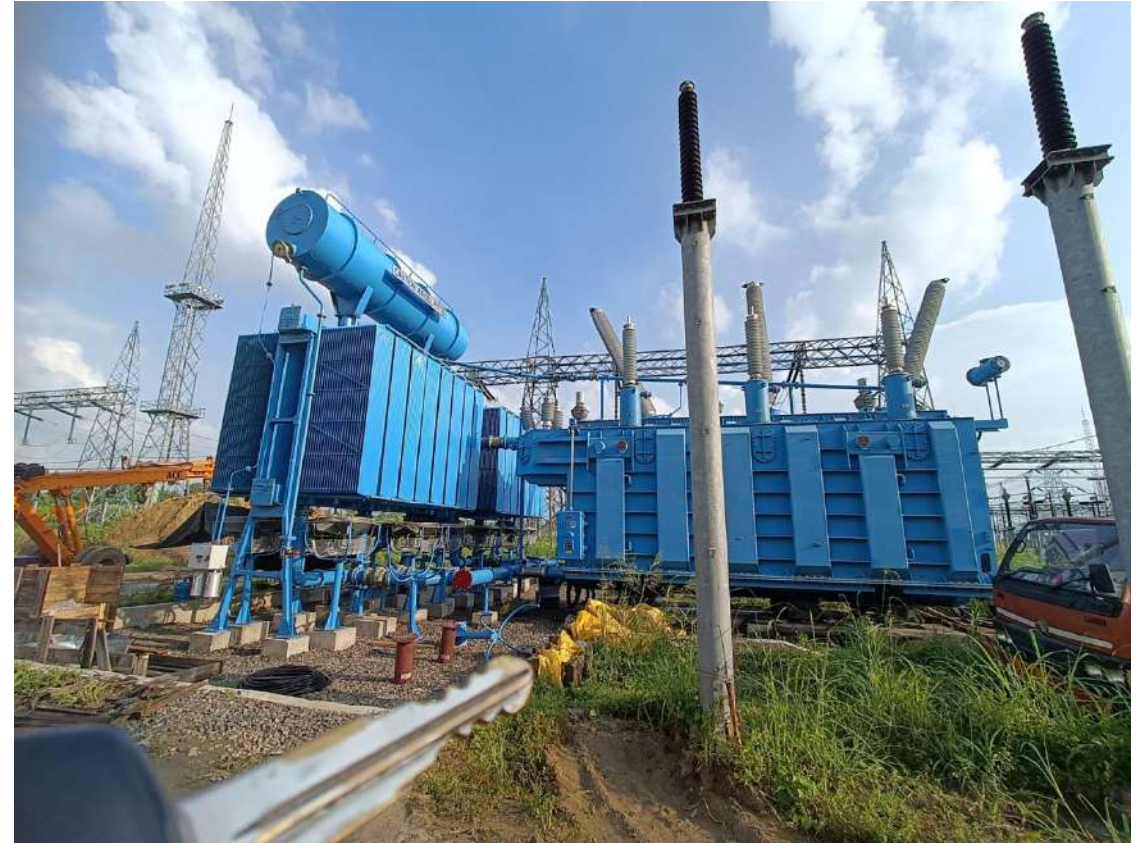
2 Nos. 200MVA ICTs Erection and Commissioning Manufacturer- BHEL FDPS – M/s GE T&D (I) Limited
