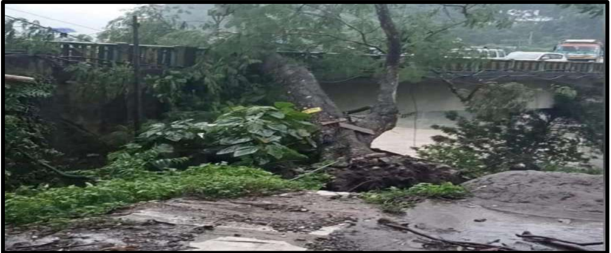
20th Mile landslide
