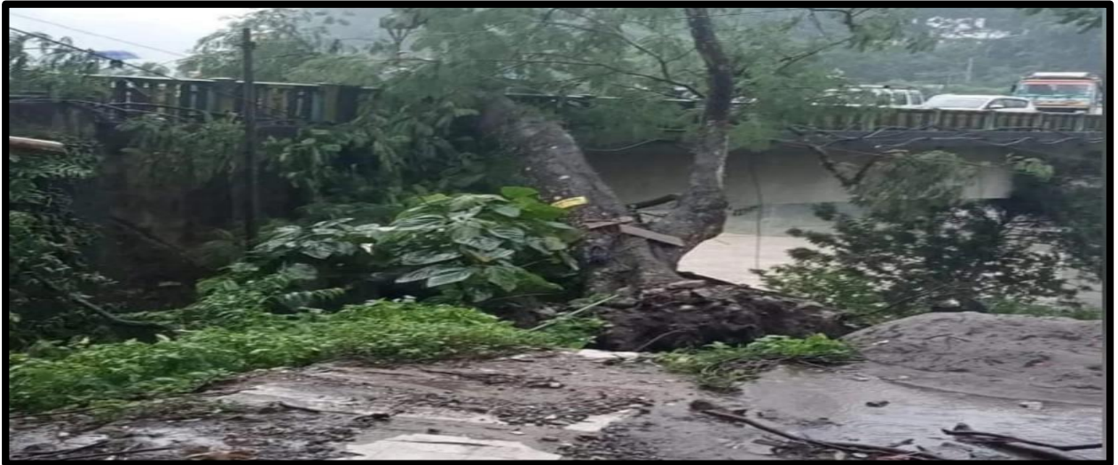
20th Mile landslide
