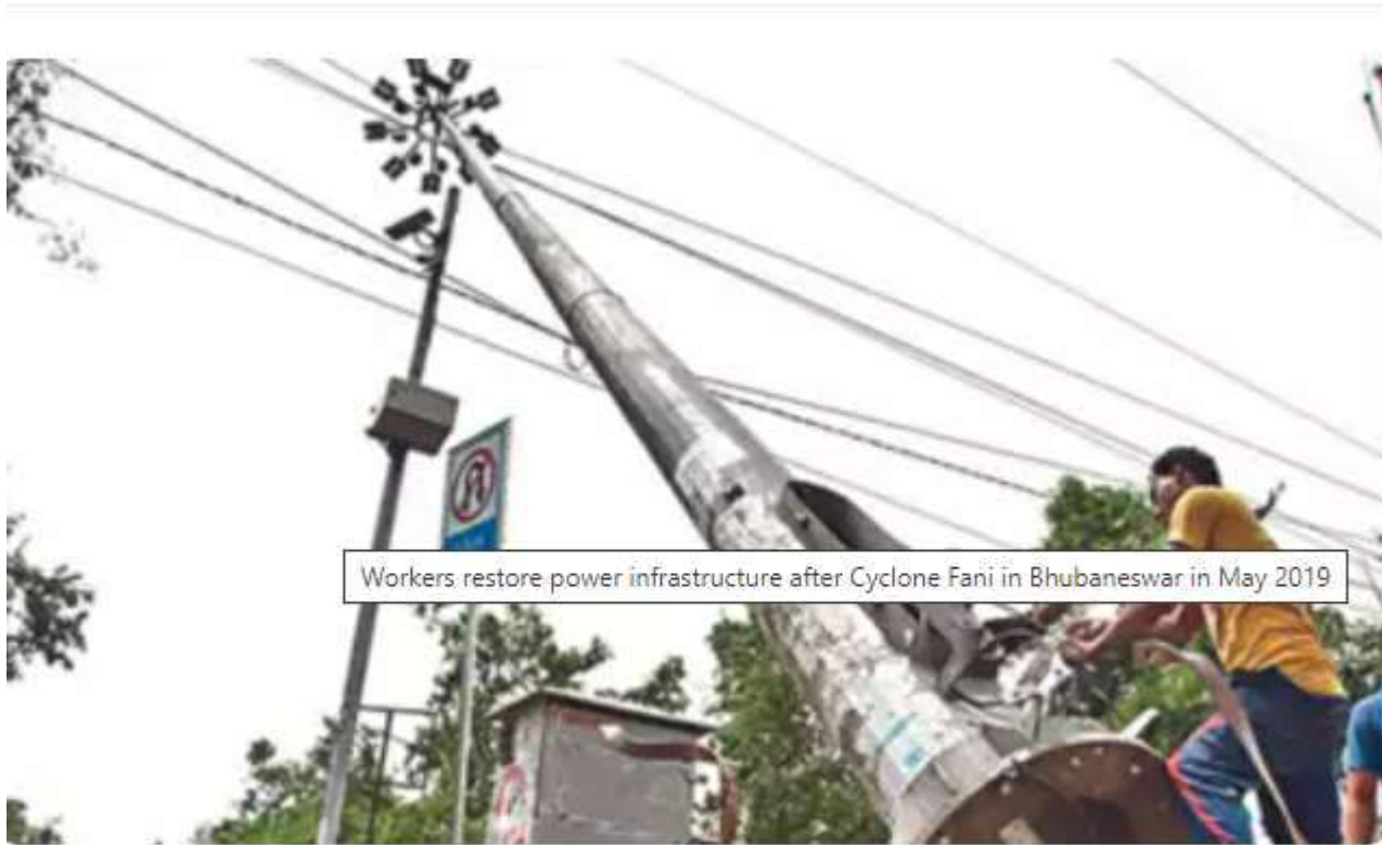
Workers restore power infrastructure after Cyclone Fani in Bhubaneswar in May 2019
