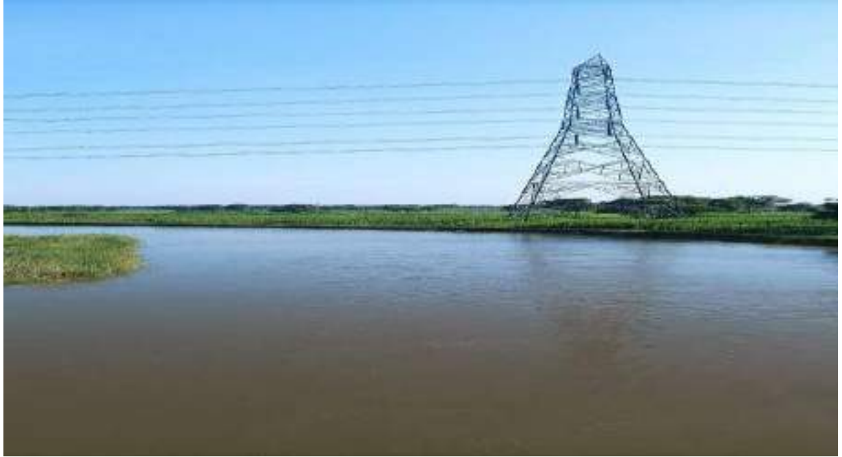
Before- Photographs of Tower no. 97
