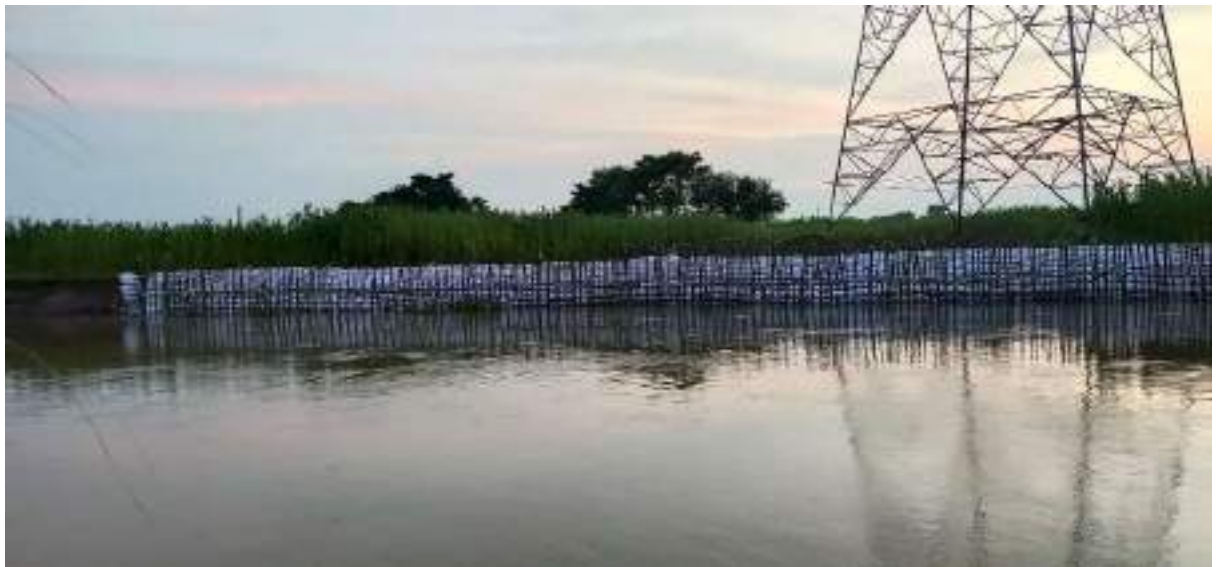
After- Photographs of Tower no. 97 (Tower protection by using Bamboo piling & Geo Bags)
