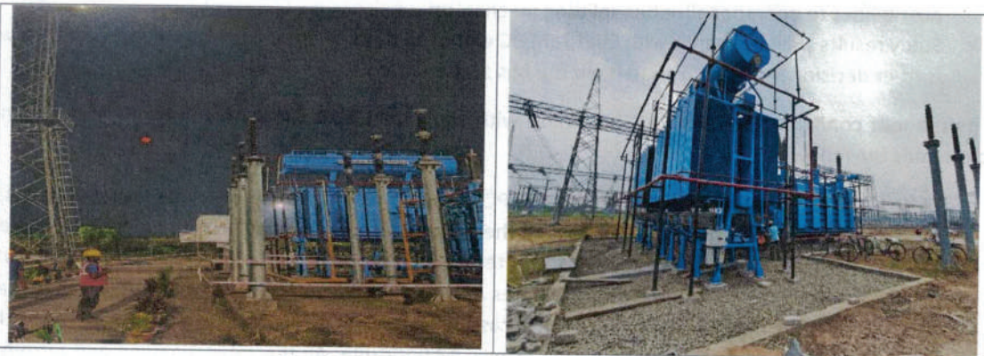
Erection works of ICT 3 & 4 completed
